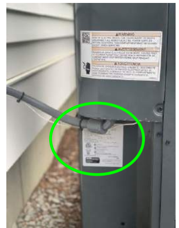
Model number and Serial number location for the outside compressor
