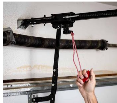
The emergency cord will automatically reengage when power is restored.
